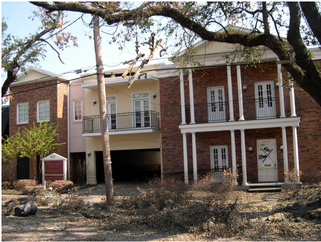
Ericksen, Krentel & LaPorte's New Orleans office on Canal Street sustained extensive first floor water damage from Hurricane Katrina. The water line is visible just below the door handle to the office building that is marked by officials' spray paint indicating the building had been searched.
